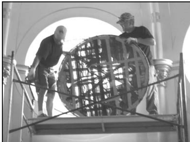
Workmen carefully remove the stained glass sanctuary windows.
