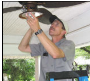
Rick Clawson installs a light bulb in a ceiling fan.
